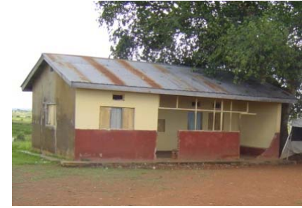
Non Functional Health facility in Amuru district: there is a need to renovate many such facilities
